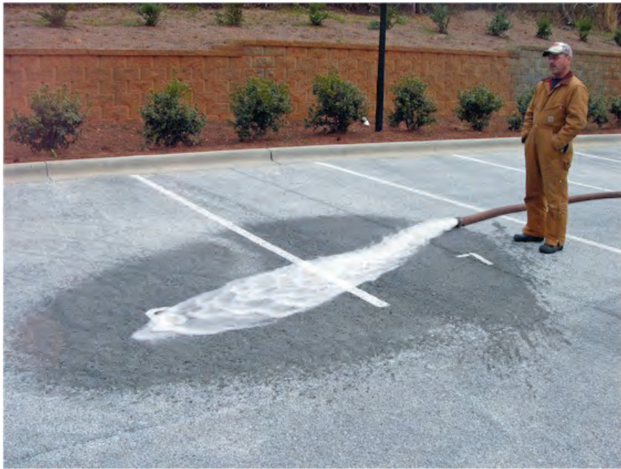
Figure 7. Wilmore Walk Reservoir filling by watering truck.
