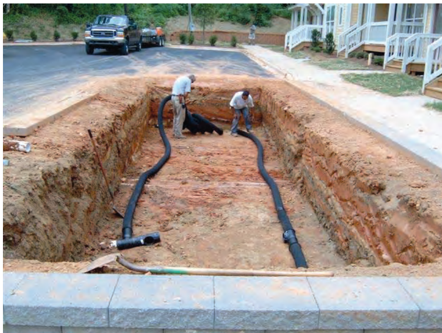
Figure 2. Installation of a bio-retention sub-drain system, Wilmore Walk
