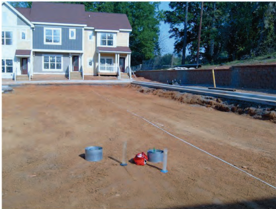
Figure 3. Native soil infiltration rate testing at Wilmore Walk.
