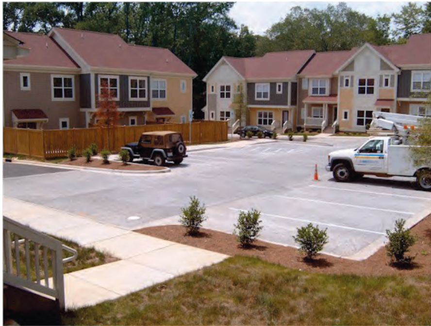
Figure 8. Wilmore Walk finished porous concrete parking lot
