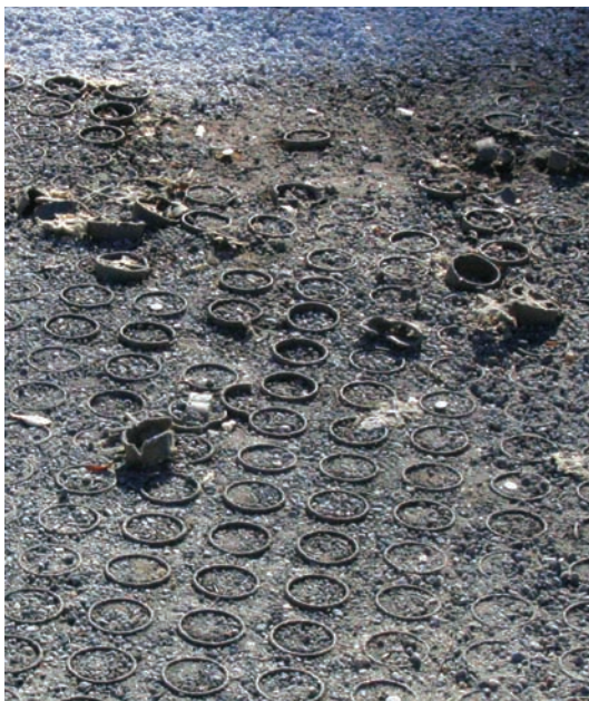
Plastic geocells are not sturdy enough to support heavy traffic, as in this Athens, Georgia, parking lot.
