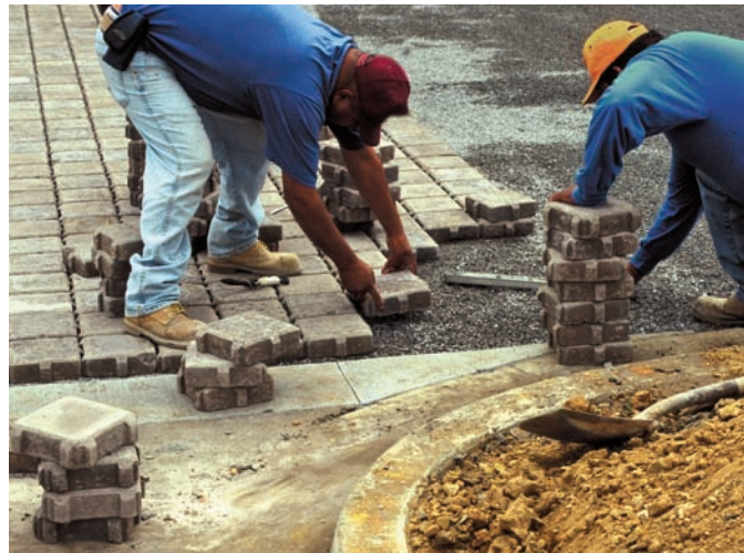
Workers install concrete blocks in a parking lot at the Robson Center in Gainesville, Georgia, above. Spacers on the blocks keep the joints open, allowing water to infiltrate. The finished installation, below, has held up well.
