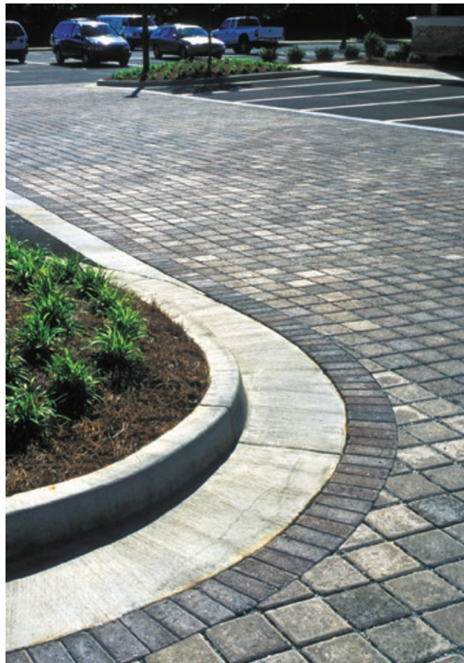
Workers install concrete blocks in a parking lot at the Robson Center in Gainesville, Georgia, above. Spacers on the blocks keep the joints open, allowing water to infiltrate. The finished installation, below, has held up well.
