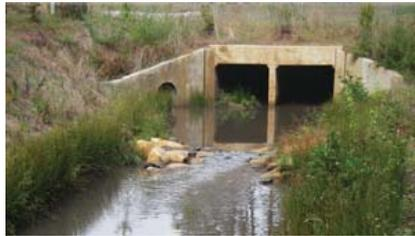
Water quality best management practices, such as wet ponds, typically have forebays with culvert inputs. Incorporating correctly sized natural plunge pools can enable a more compact design for velocity attenuation. This allows a greater "stilling" effect for more efficient pollutant removal. Photos: Estes Design Inc.
