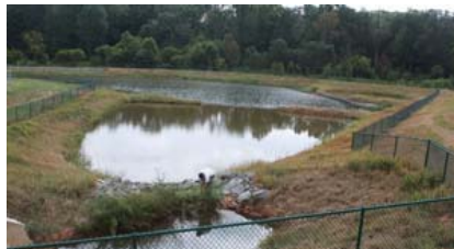
The natural plunge pool design methodology can also be used to transition steep grades by incorporating the methodology into step pool design.
