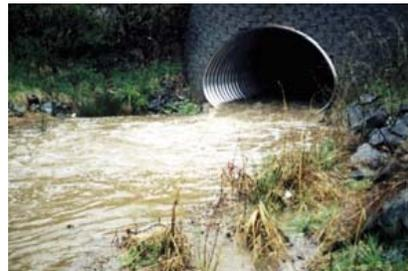
Culvert outlets with submerged tailwater conditions typically exhibit a variation in designed pool geometry from their counterparts with free-falling jets or supported jets.
